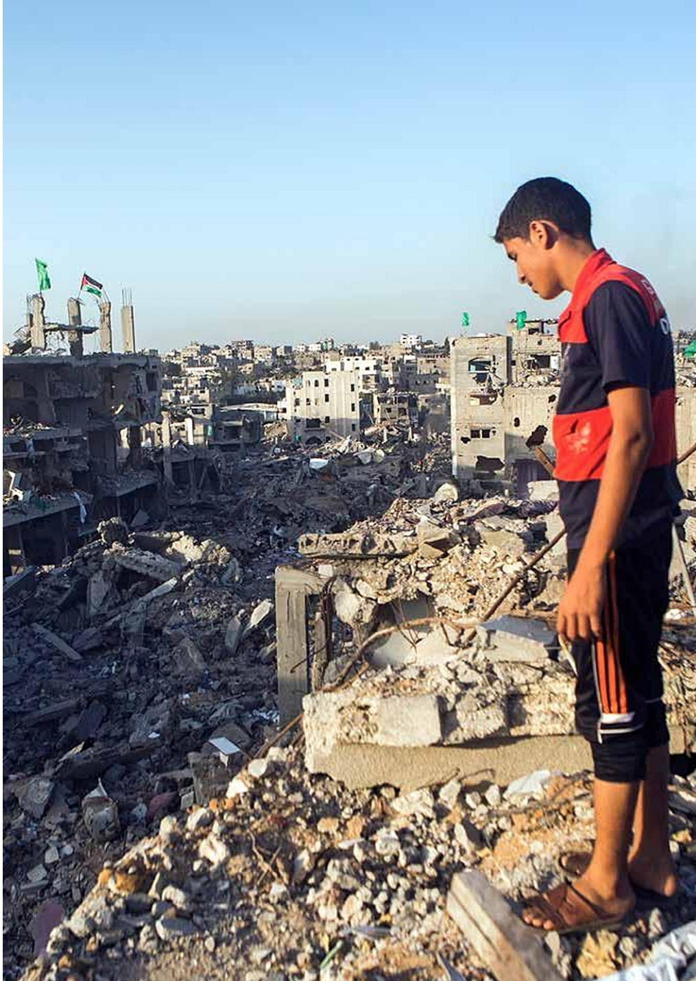
photo: Activestills.org. A Palestinian youth stands on the roof of a destroyed house September 4, 2014 in Shuja'iyya neighborhood, east of Gaza city, which was heavily attacked during the Israeli offensive.
